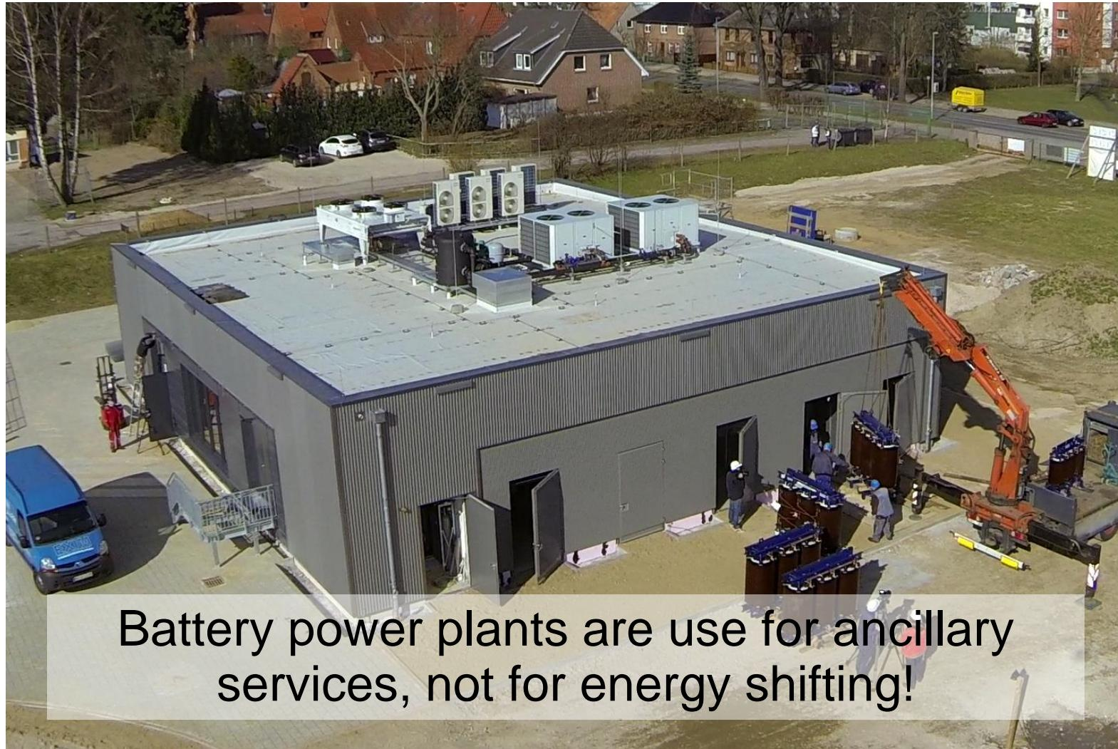
Battery power plants are used for ancillary services, not for energy shifting!
